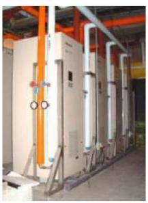
Solar collectors placed on the roof. Storage tank placed in the mechanical room: The sun heats the water as it passes through the collector and then is circulated to a storage tank.
