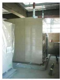
Ice storage systems make ice during the night when electric utilities charge less for energy. The ice supplements or even replaces mechanical cooling during the day and can result in significant operating cost savings
