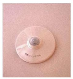
Ceiling daylight sensors: it is automatically switched on or off when day lighting reaches a certain level. Ceiling occupancy sensors: it is automatically switched on or off with sensing the occupant
