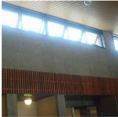
Interior view of the upper windows for air exhaust (Bathhouse)
