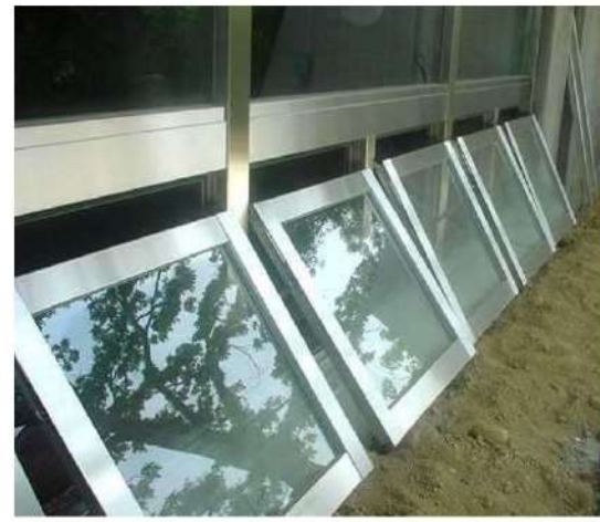
Exterior view of the lower windows for air supply (Bathhouse)
